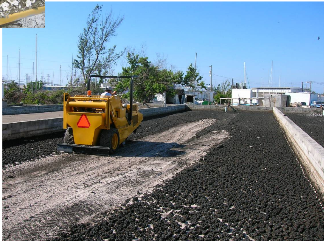
Using a small hole sized screen, the crust of the sediment can be loaded while the fines are returned to the bed.
