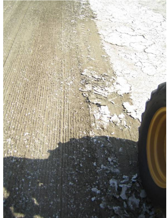
Using a small hole sized screen, the crust of the sediment can be loaded while the fines are returned to the bed.
